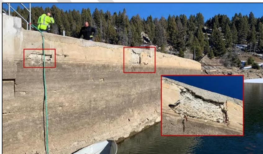
Upstream view of parapet wall condition (near spillway)
